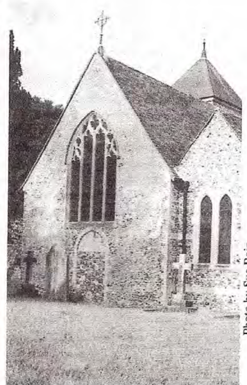
Exterior view of the Church of St. Lawrence the Martyr, Godmersham, from the east showing the roof valley in need of major repair.
